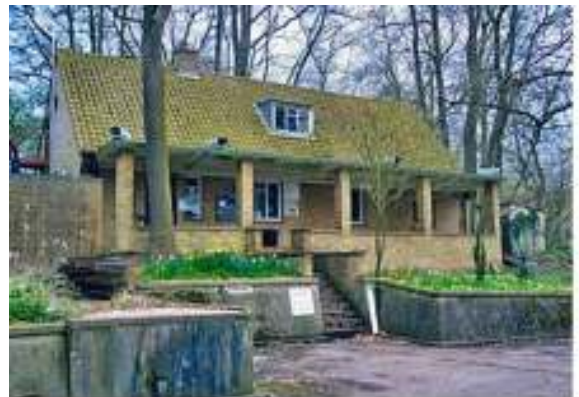
This is the entrance to the bunker. Disguised to look like a farm house, it is in fact constructed of four foot thick concrete.
